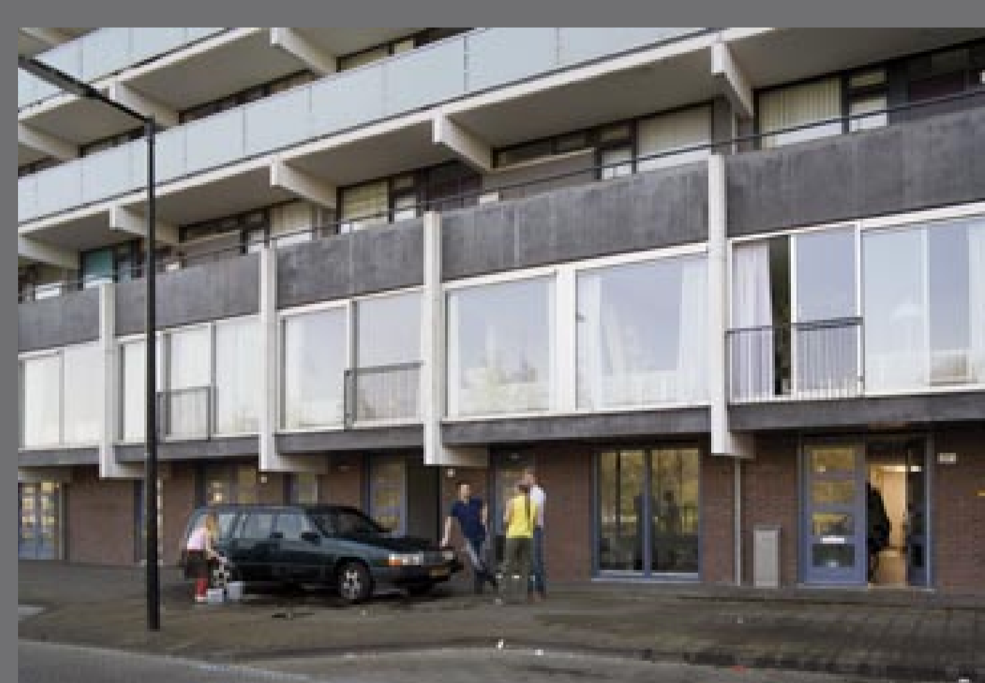
connection to the street studios in groundfloor, living space in the former covered street (1 st floor)
